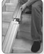
**Step 7:** Install rail brackets by loosening the screws and snapping each bracket edge into the slot, or slide the brackets on from the top of the rail.
